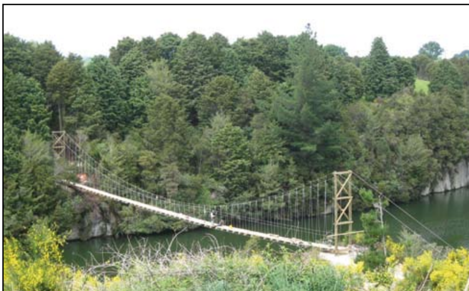
The Waikato Trail bridge design will be replicated for the Otara River bridge. Construction begins in March.
