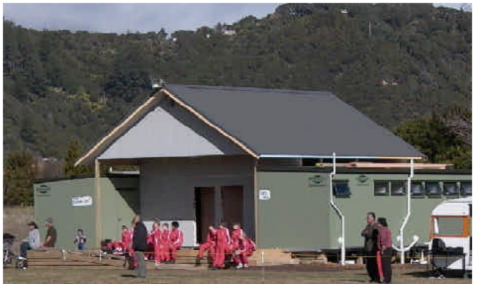
The brand new toilets and changing rooms were put in place at Te Whanau A Apanui Area School in time for the Tai Mitchel Tournament.
